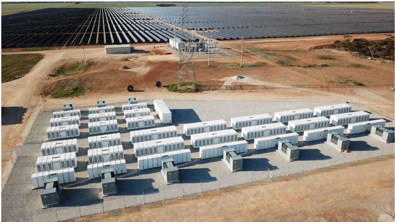
Large scale battery storage at Gannawarra, Australia.
