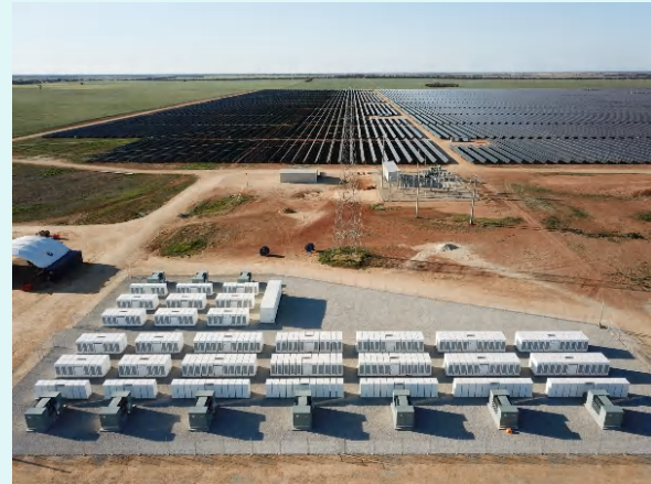
The large battery at Gannawarra, underpinned by EnergyAustralia, is an example of the changing technologies shaping the energy system.
