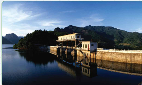
Guangdong Huaiji Hydro Power Station
